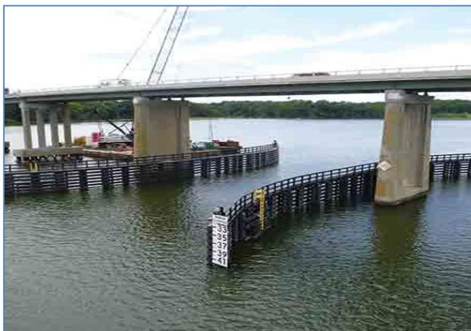
Picture 4: Fenders for collision protection
