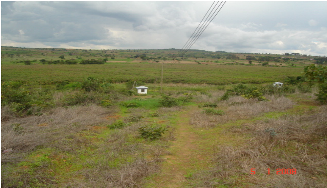
Fig 6.3: Two pumping Station (Borehole) at Lwiche valley
