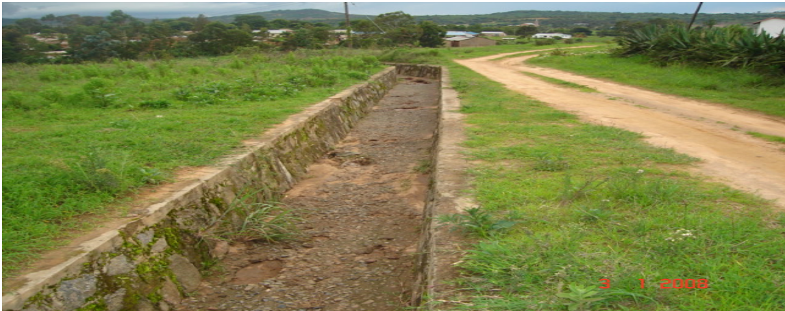
Fig 6.1: Storm Water Stone Pitched Channel.
