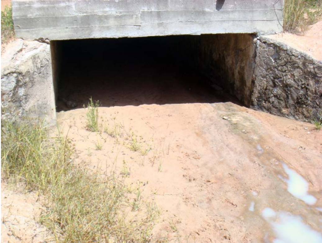
Fig 6.2: Drainage Structure at One end of the Runway
