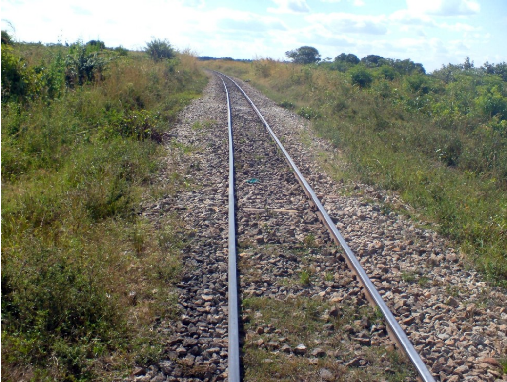
Fig 4.2: Railway Line adjacent to the airport
