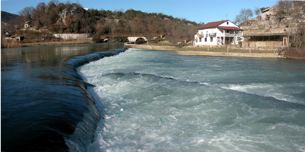
Figure 1: Mlade/Trebizat River downstream of Klokun bridge (view direction: upstream)
