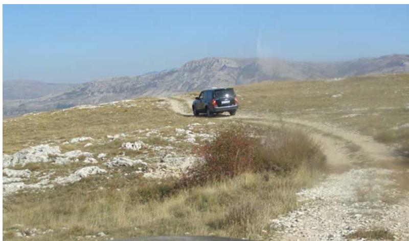
Picture 4.9 Macadam road to wind farm Mesihovina
