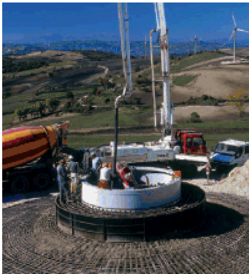
Picture 3.6 Typical foundation for a wind turbine
