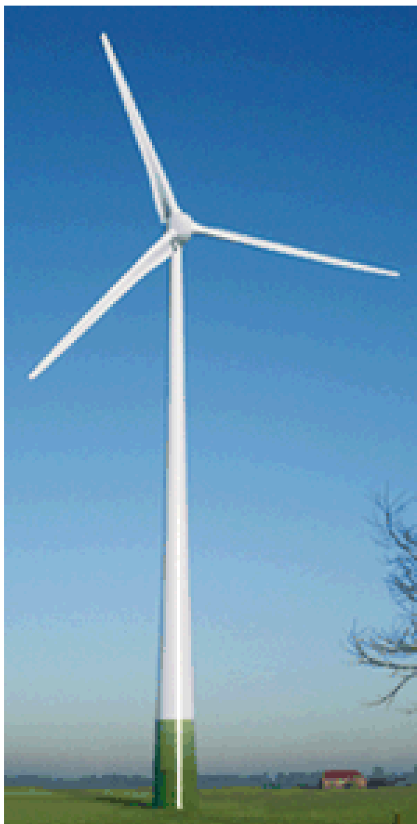
Picture 3.4 Typical 2 MW wind turbines Enercon E-82
