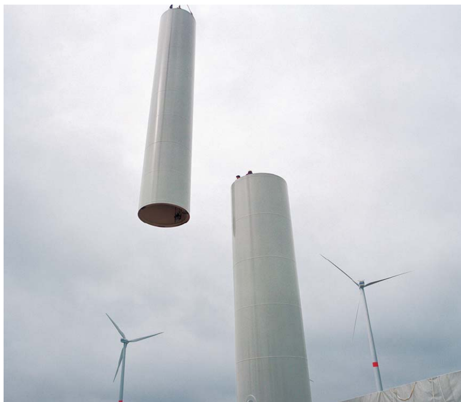
Picture 3.7 Mounting of the wind tower
