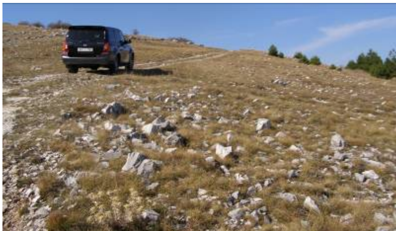
Picture 4.8 Macadam road to wind farm Mesihovina
