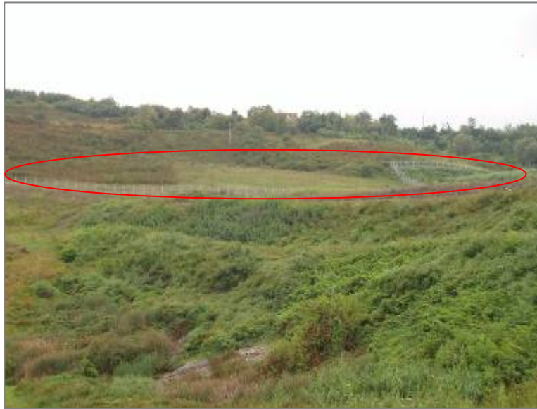
Photograph no. 17 The view on the landfill from direction of accessing road
