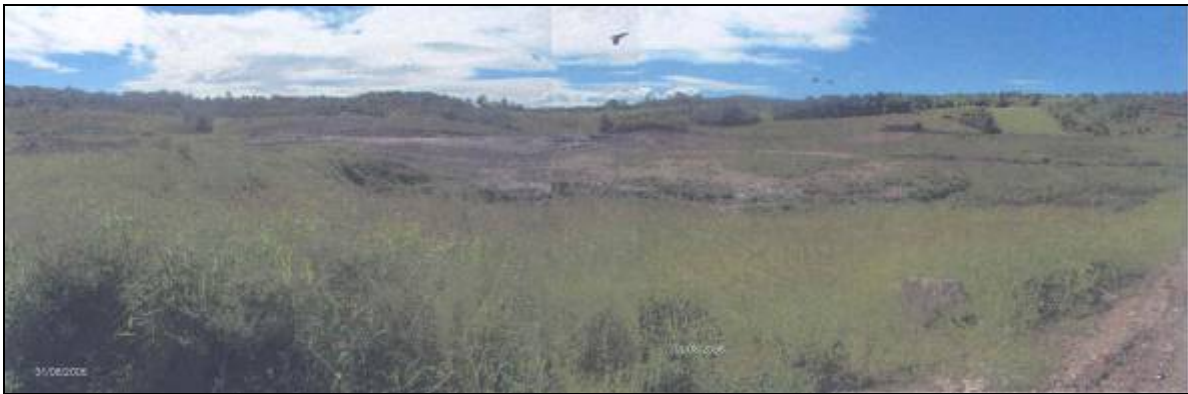
Picture no. 3. The landfill Ramići, the view on the land south from wasteland
