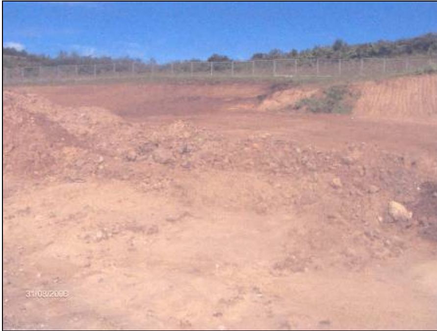
Picture no. 6 the Ramići landfill, the view on the canal on the landfill entrance
