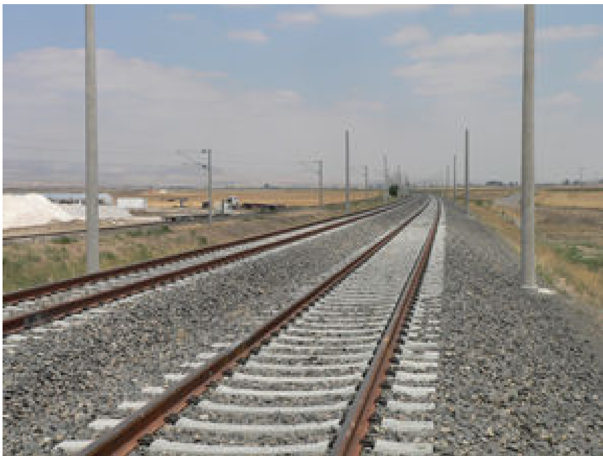
Figure 6. A typical view of a newly constructed dual-line.
