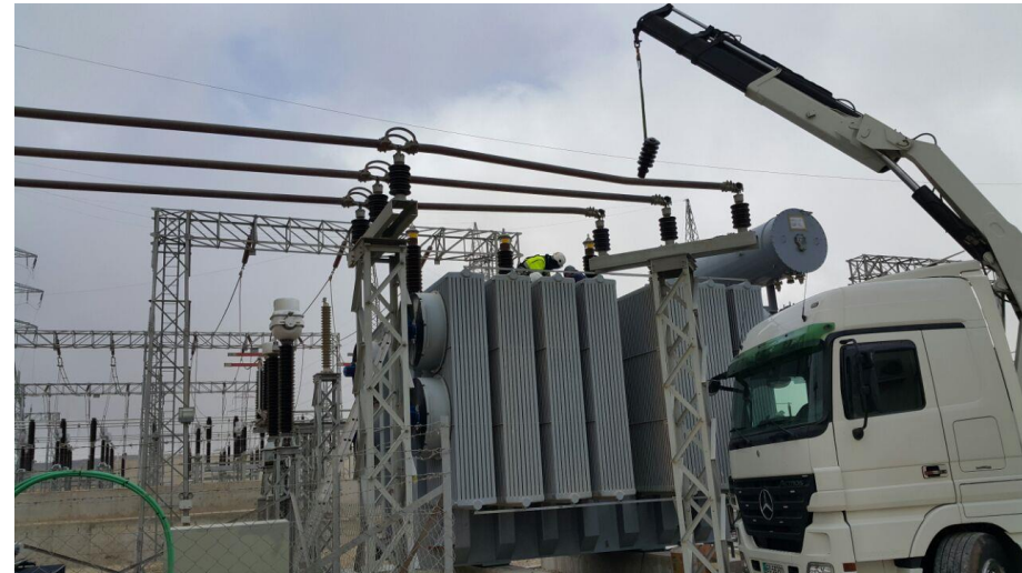
Transformer Transport and Installation
