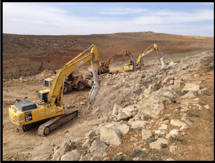
Foundation excavation
