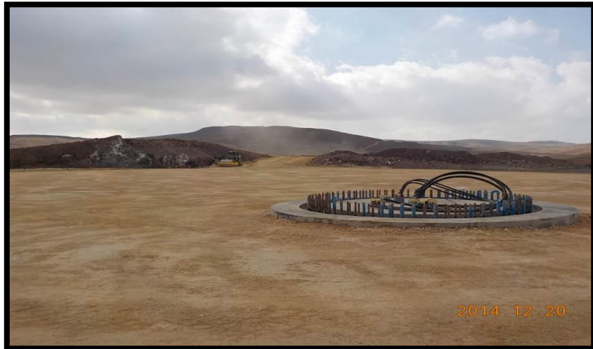
Backfilled foundation
