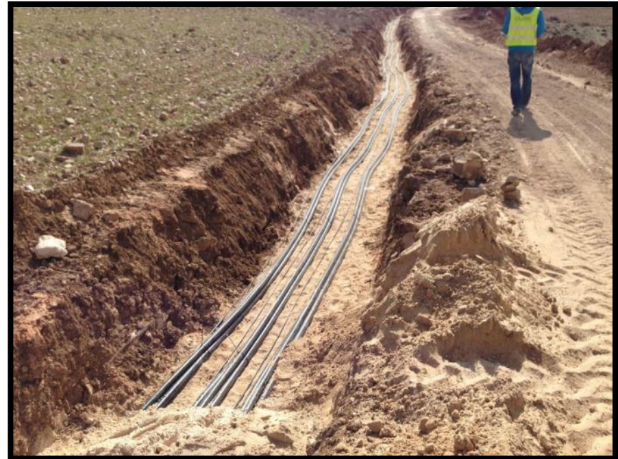
33kV cable works
