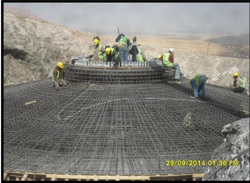
Foundation reinforcement works
