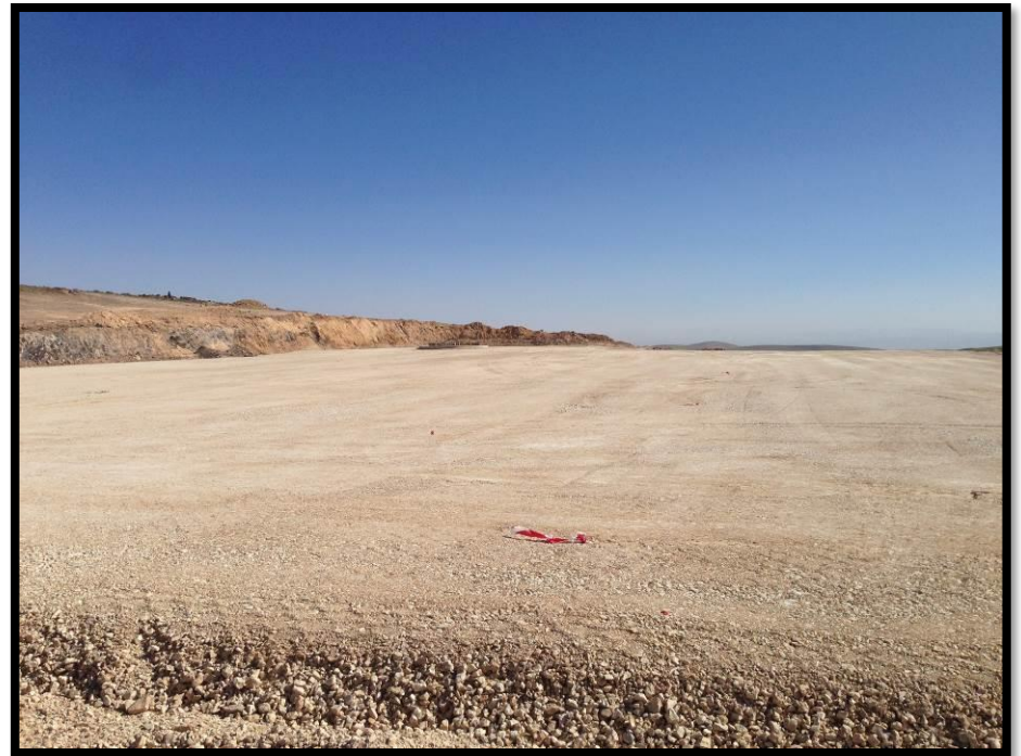
Completed crane pad
