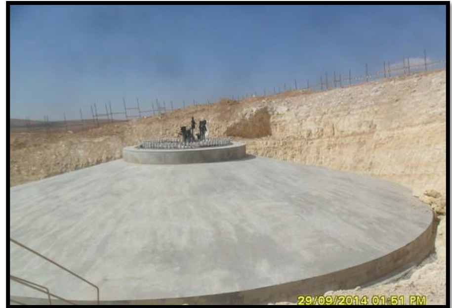
Completed Foundation ready for backfilling
