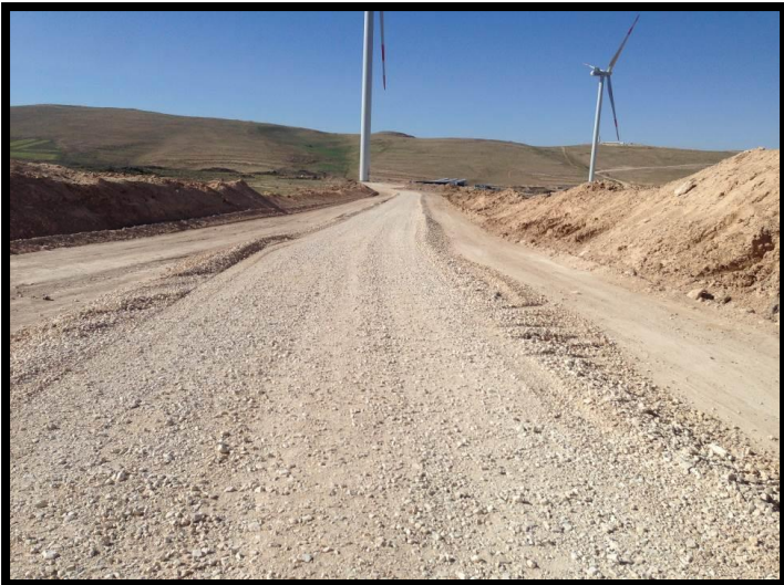
Completed site road
