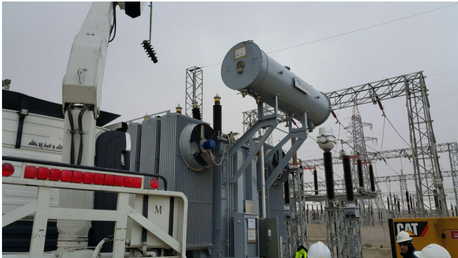
Transformer Transport and Installation
