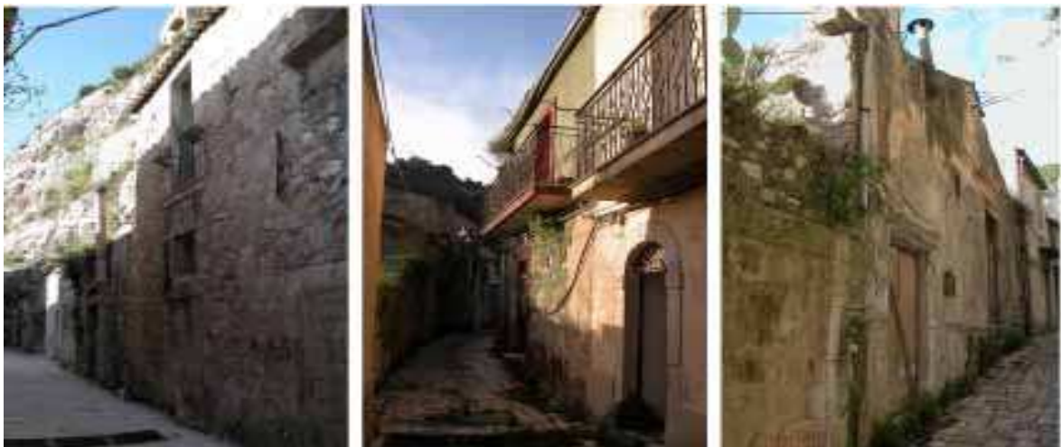
Figure 15 - Views of Via Velardo in its current condition
