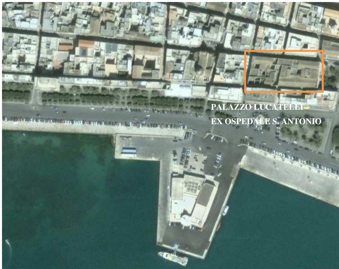
Figure 8 – Aerial view and localization of Palazzo Lucatelli
