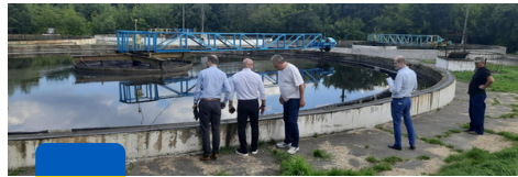
Field visit to Khmelnytskyi water treatment plant, Ukraine, August 2025
