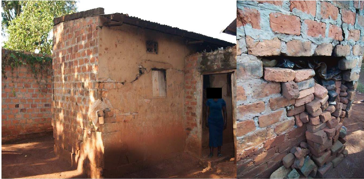
Houses in Malindi, village closest to the Bujagali Dam
