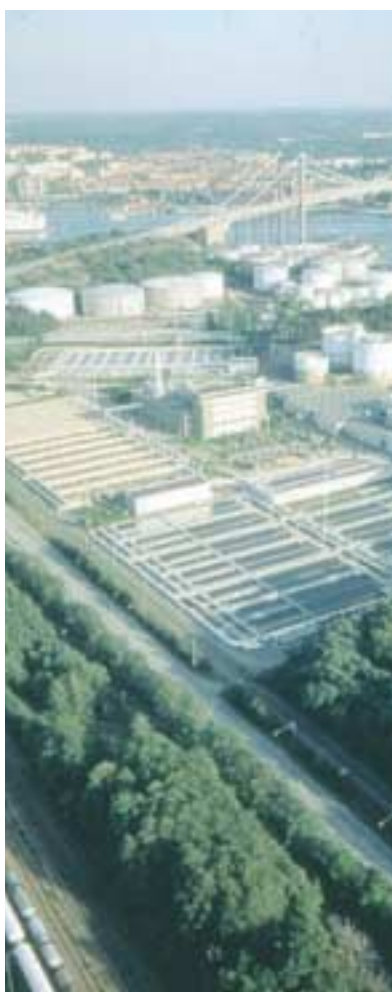
Wastewater Treatment Plant, Stockholm, Sweden
