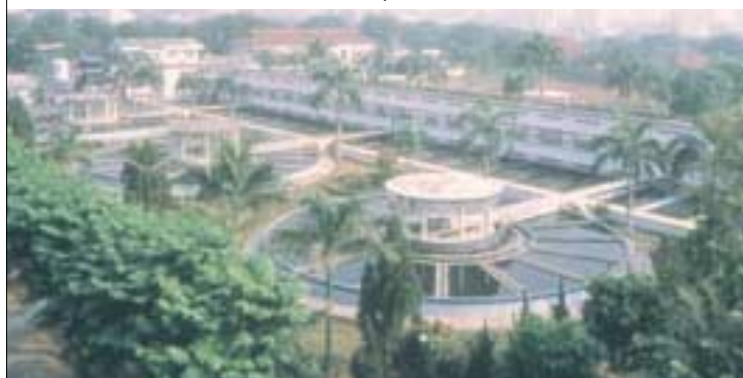
Water treatment plant, Jakarta, Indonesia
