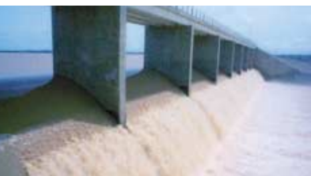
Water Infrastructure, Ouagadougou, Burkina Faso
