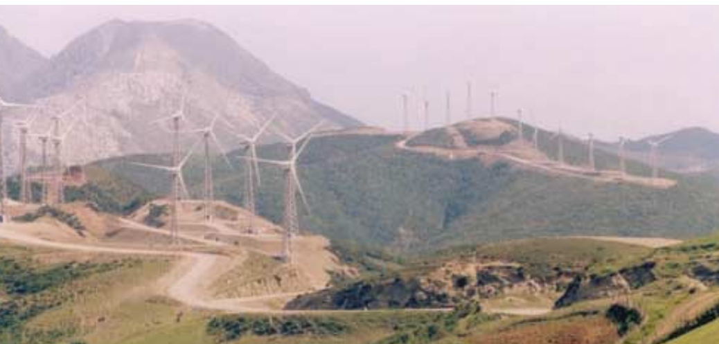
Wind Farm, Tetouan, Morocco
