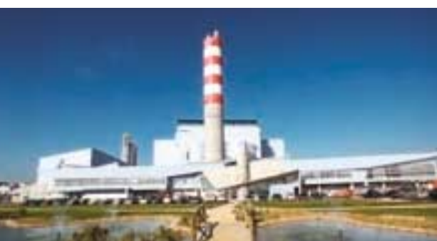
Solid Waste Treatment Plant, Portugal
