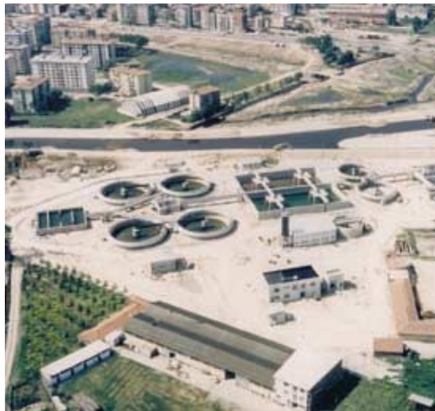
Wastewater Treatment, Turkey
