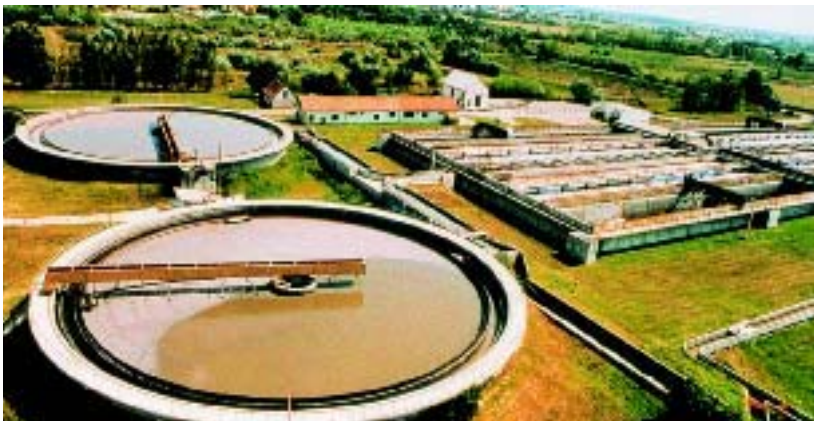
Waste water Treatment Plant, Debrecen, Hungary
