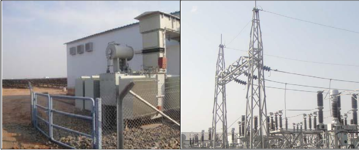
Figure 3.23. Sample Transformer Station (Step-up) and Switchyard Photos (Source: Asia Development Bank, September 2015)
