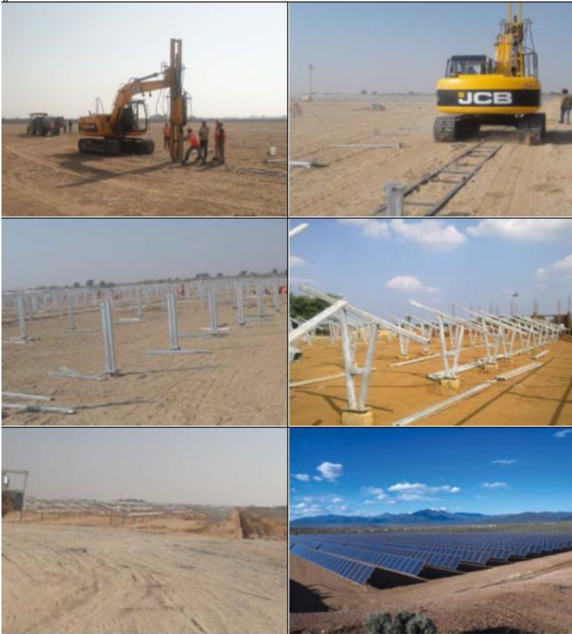
Figure 3.20. Sample Photos Showing Assembling Phases of Solar Panels (Source: Asia Development Bank, September 2015; IFC, February 2012)
