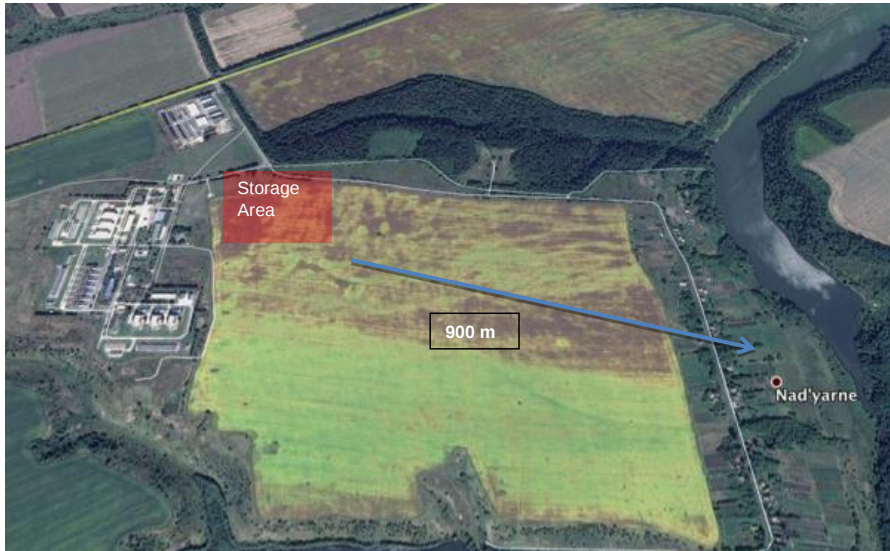
Figure 4-8 Storage Area of Section-1
