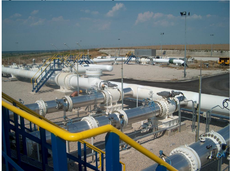
Figure 6.6 Typical (border) Metering Station.
