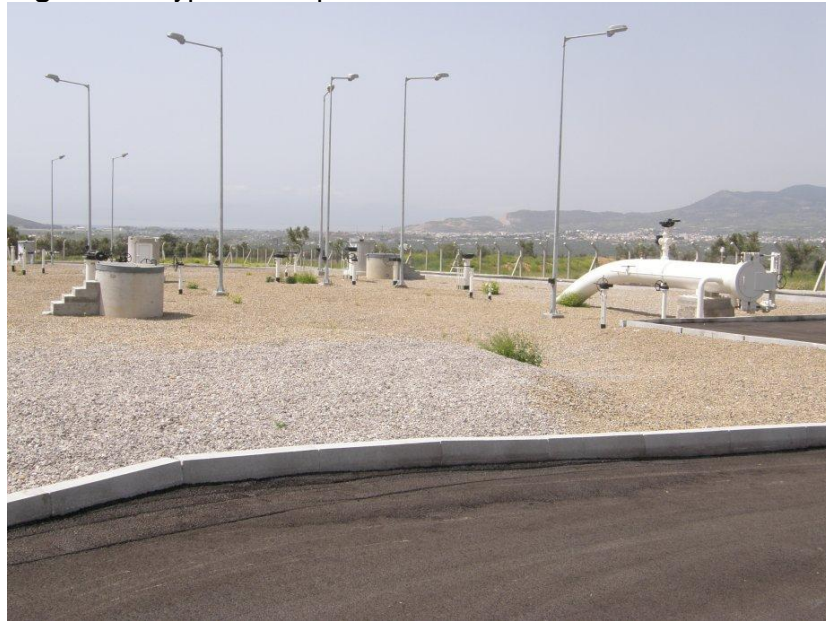
Figure 6.7 Typical Scraper Station Installations
