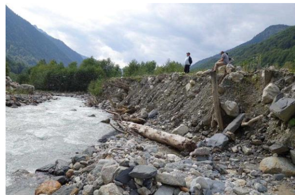
Nakra River – at Nakra village – remains of solid material transported by Lekverari torrent following landslide in 2011 – and which blocked the Nakra Illustrates the depth of material that blocked the river
