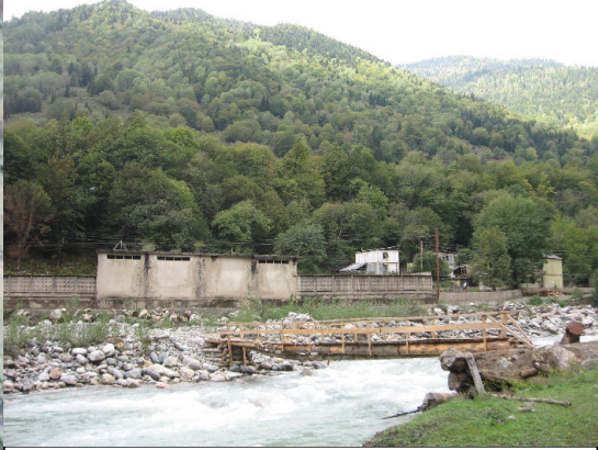
Footbridge at Upstream End
