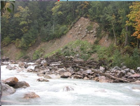
Localised Bank Slip - Left Bank
