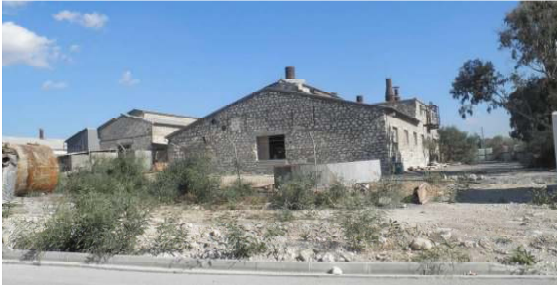
Picture 4. 6: Slop oil and Oily water processing unit (now abandoned)
