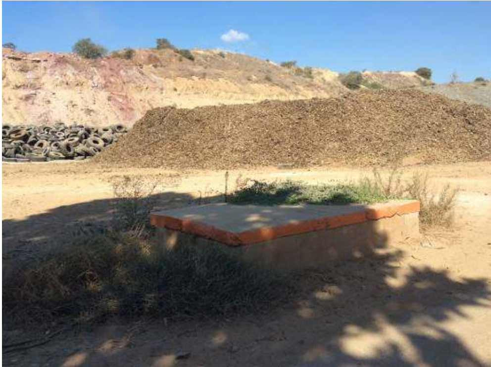
Picture 4.20: Pumping station of South Stream south of the proposed tank farm
