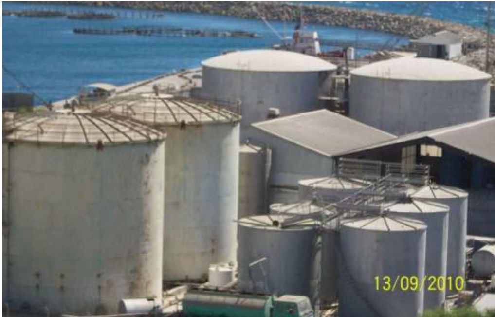
Picture 4. 9: Ecofuel installations, used oil processing facilities
