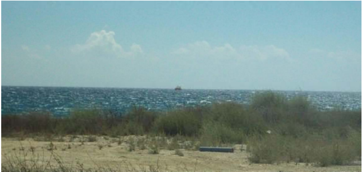
Picture 4. 11: EAC's Single Point Mooring, Vasilikos bay
