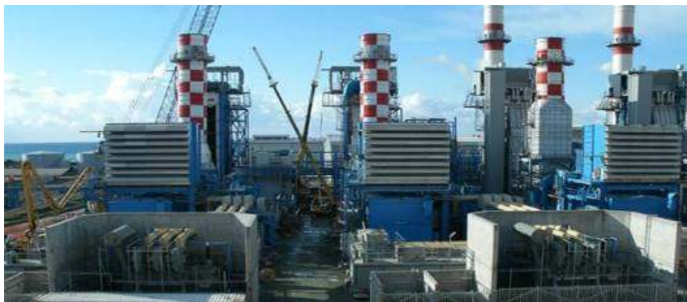
Picture 4. 1: EAC Vasilikos Power Station
