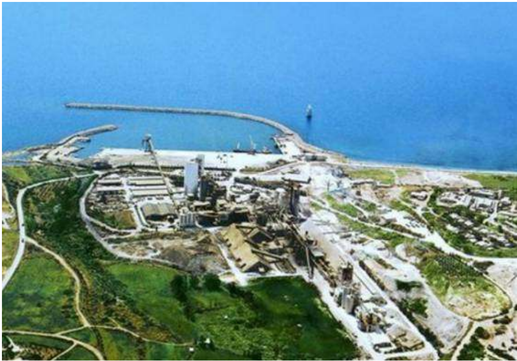
Picture 4. 3: View of Vasilikos Cement Works
