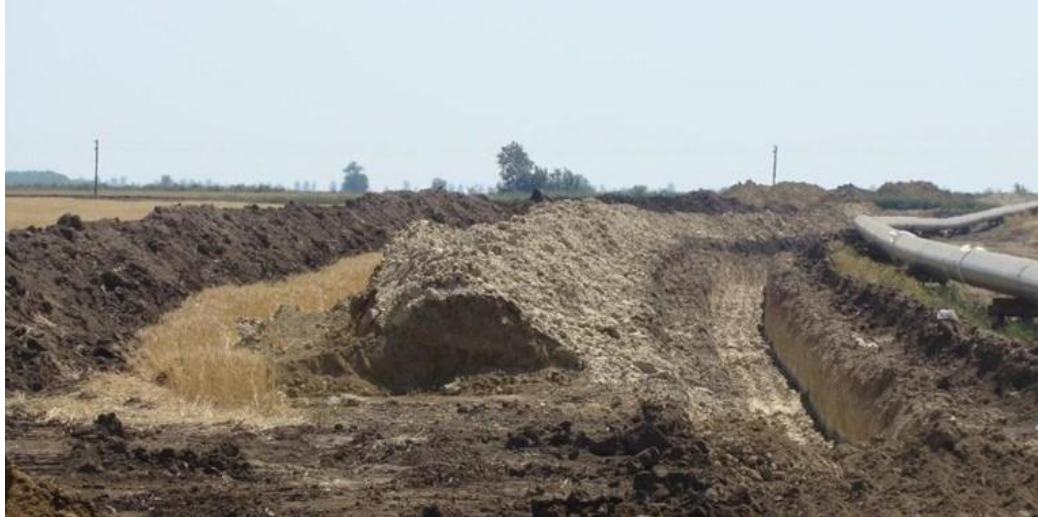
Figure 2.2 Illustration of a typical working strip.
