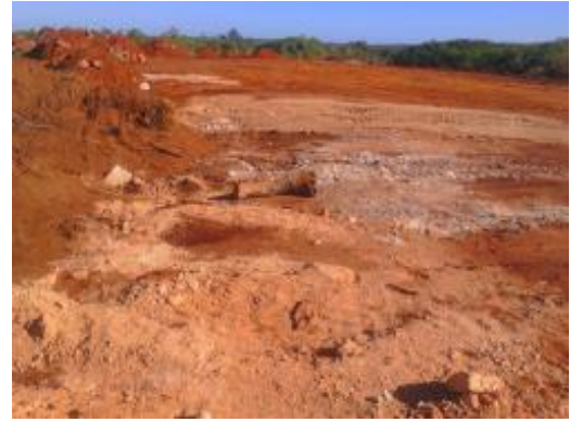
Opened up earth crust points within and around the project site examined for possible archaeological artifacts
