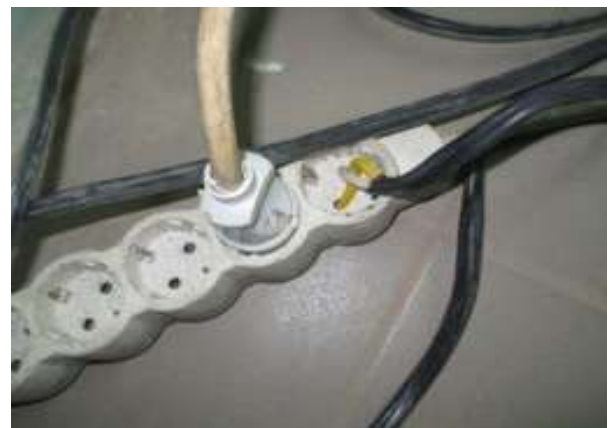
Figure 14: Electrical equipment usage at Peremoha station
