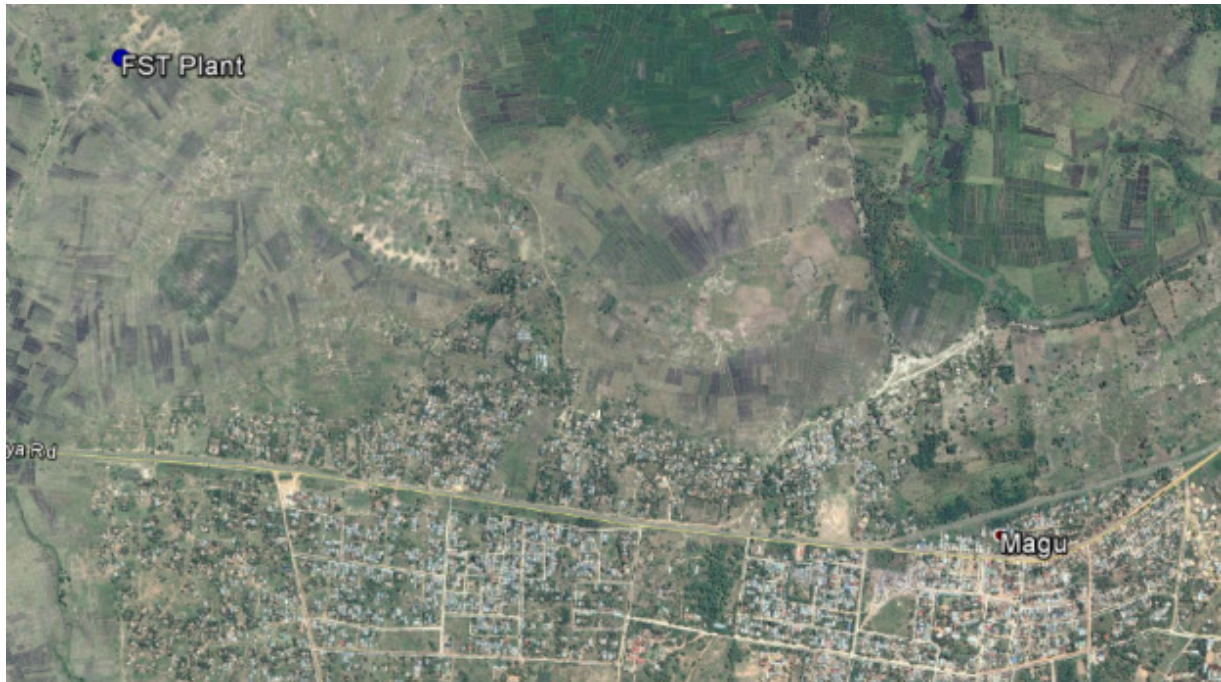
Figure 2-2. Proposed land for construction of the faecal sludge treatment plant for Magu town
