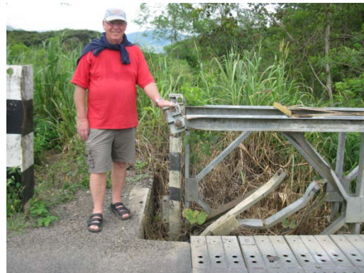
Impact damage to truss member
