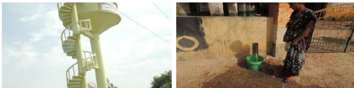
Overhead tank and tap water facility in village
