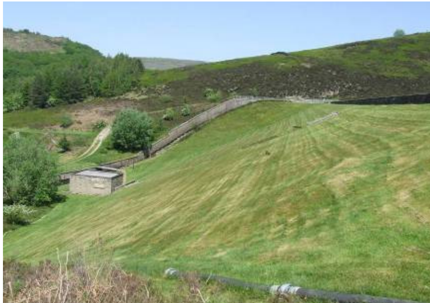
Plate 2 Reservoir embankment looking north.
