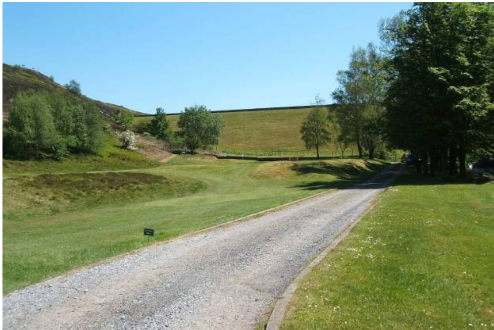
Plate 4: A view of the reservoir dam from the golf course
