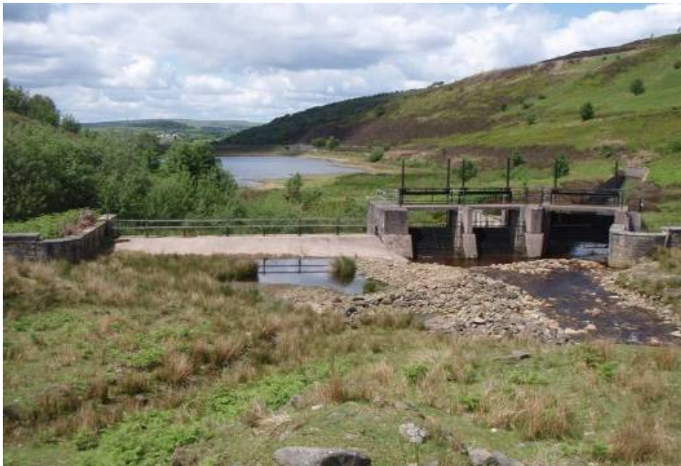
Plate 8: View looking west showing inlet structure with reservoir beyond
