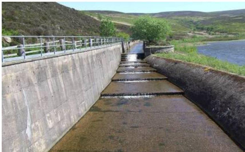
Plate 3: the bywash channel and spillway (on right) from the reservoir.
