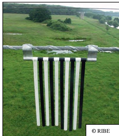
Figure 7-1: Black and white, rigid plastic pieces that swing on a rod attached at both ends to ground wire or conductor
