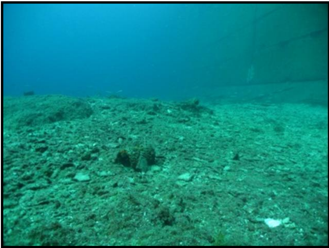
Figure 2-3 View of aggregates accumulated in the bottom of the platform
