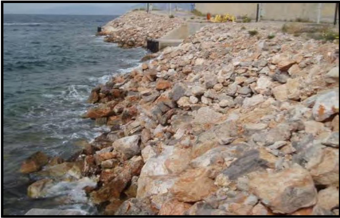
Figure 2-5 Western Part - Inadequate armoring along the western part with varying gradient of materials
