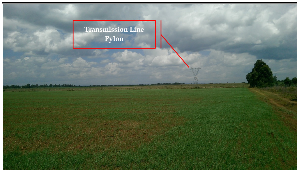
Figure 7.8 View of the Turkwel- Lessos Transmission Line
