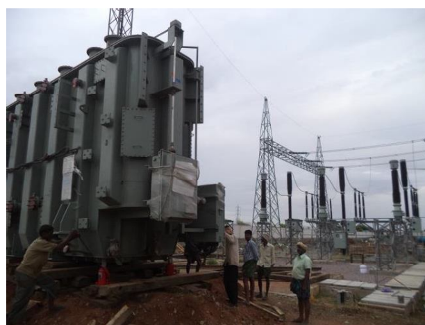
Photo 3-6: A view of construction works going of proposed 1*100 MVA transformer at Suzlon 132/33 kV Pooling Sub-Station
