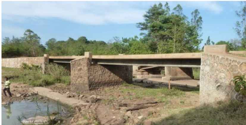
Figure 158 – Bridge made with cement culverts
