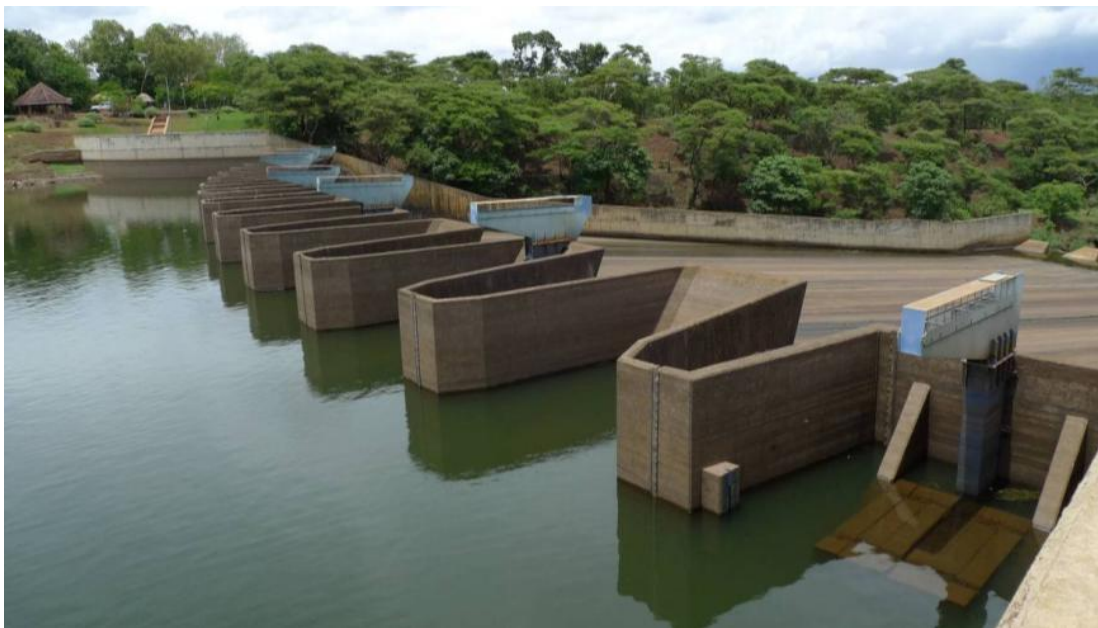
Figure 4 – 5 m Fusegates system used in Kamuzu Dam II raising
