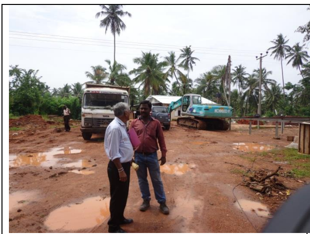
Figure 17 general site after removal of soil
