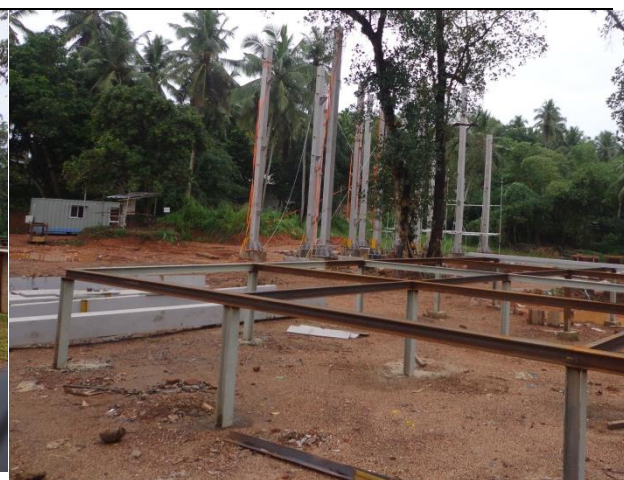
Figure 18 Construction in progress
