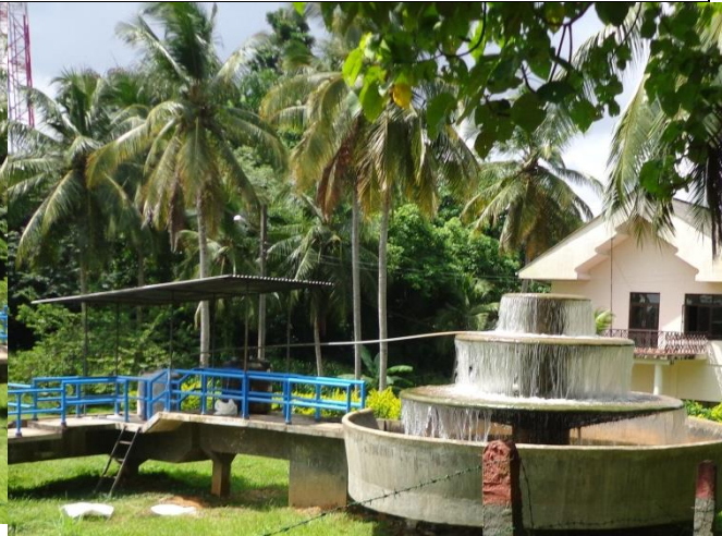
Figure 13 Aerator at the BOI facility
