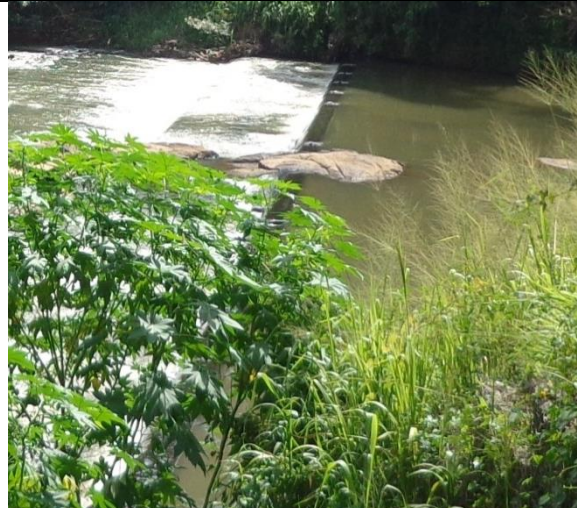
Figure 10 water intake & weir at the Maha Oya
