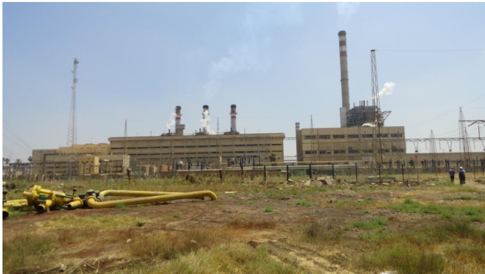
Photo 5-1: Landscape at the vicinity of Damanhour Power Plant
