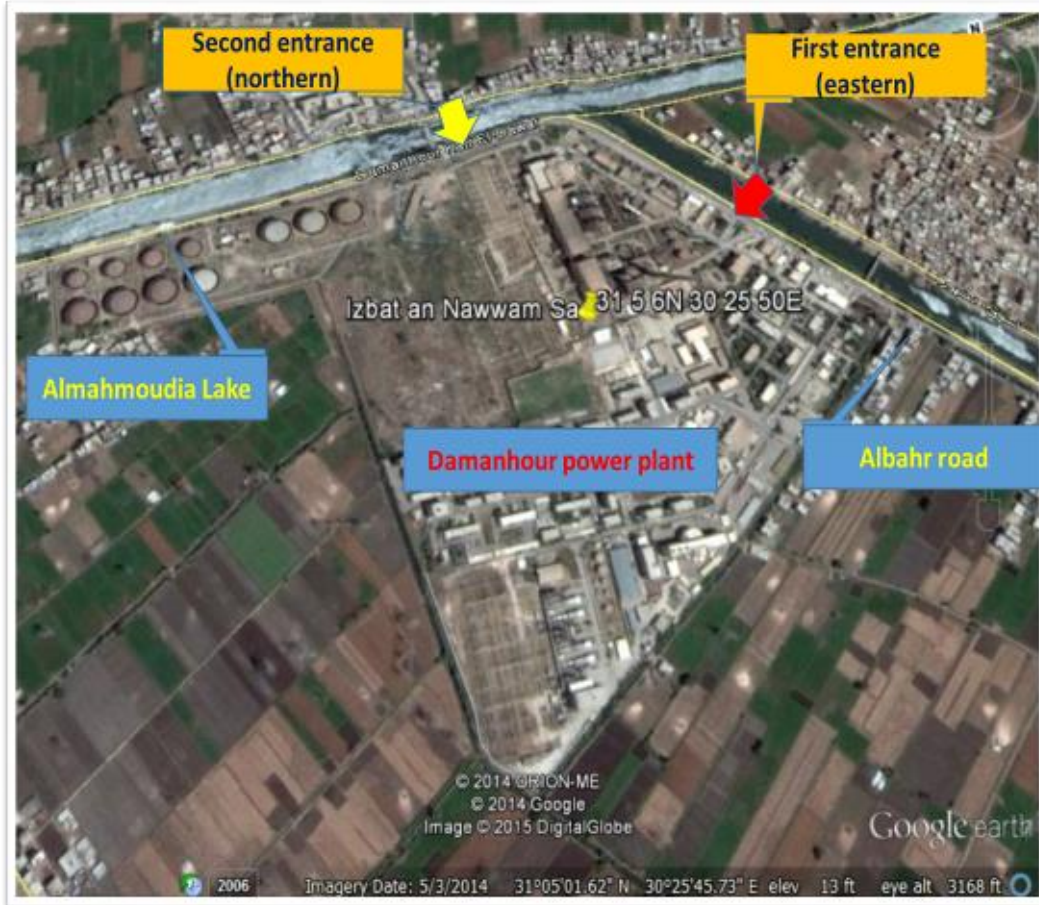
Figure 5-30:: Entrances to Damanhour Power Station
