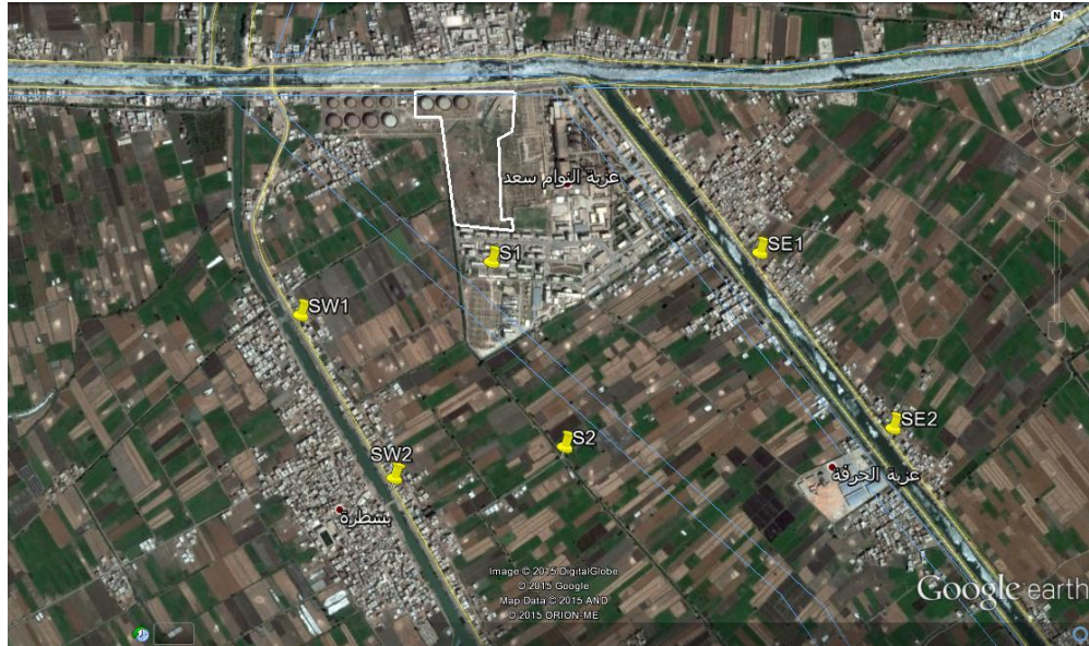
Figure 5-3: Measurement Locations outside of Damanhour Power Plant
