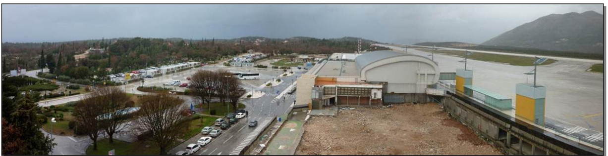
Photo A.1-2. The current appearance of the Dubrovnik Airport (view of the demolished building "C" terminals, parking)
