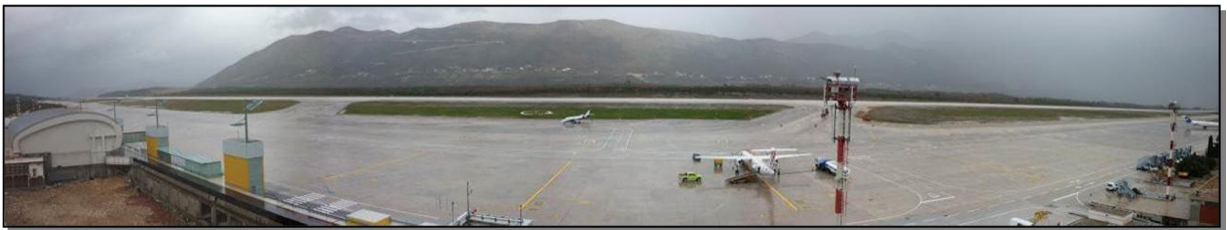
Photo A.1-1. The current appearance of the Dubrovnik Airport (apron, taxiways and runway)
