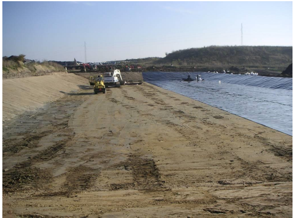
Figure 2.3 Construction of clay liner and installation of HDPE-liner
