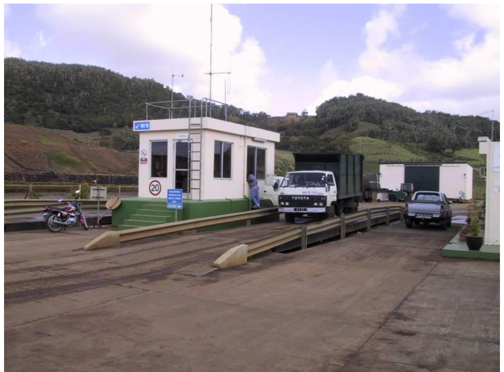
Figure 2.2 Electronic weighbridge for trucks delivering waste to the landfill
