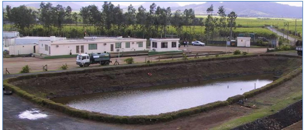
Figure 2.1 Reception area with weighbridge, buildings and leachate pond
