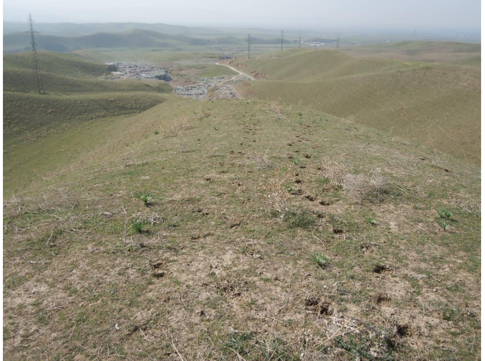
Figure 1.2 View over the proposed site for sanitary landfill in upper part of valley partially occupied by Jalal-Abad dumpsite (the dumpsite is visible in the background)
