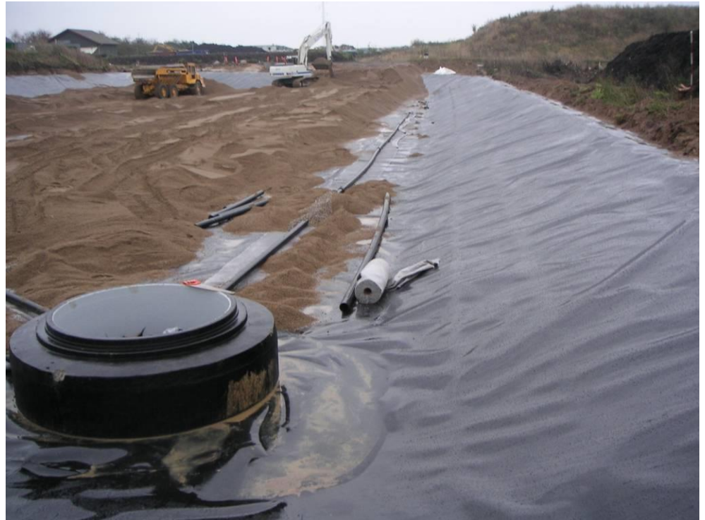
Figure 2.4 Installation of drainage layer on top of the HDPE liner
