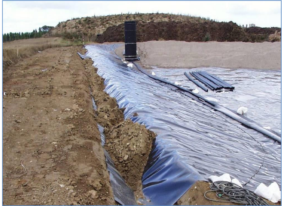
Figure 2.5 Construction of waste disposal cell, with bottom clay layer, HDPE liner on bottom and slopes, and a leachate collection well at the lowest point of a landfill cell
