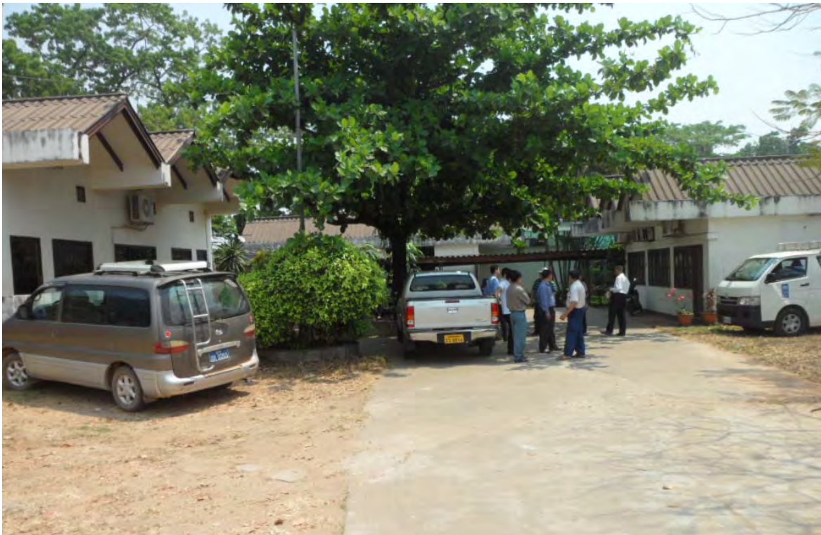
Photo 3. Existing building at the IMMC compound
