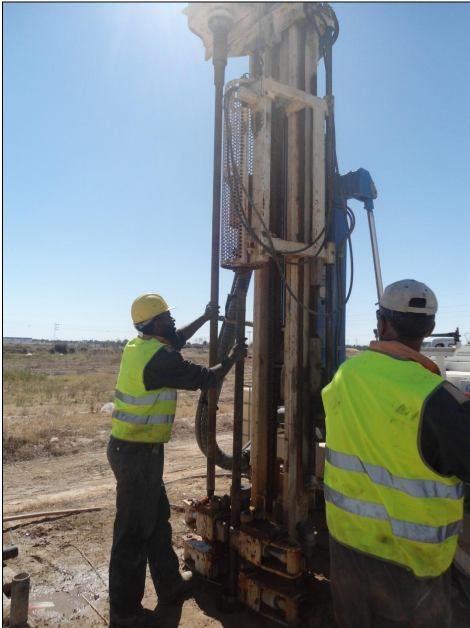
Figure 4 : Coring works on the site of the projected gas treatment plant (photo taken on April, 18th 2013 at Ghannouch)
