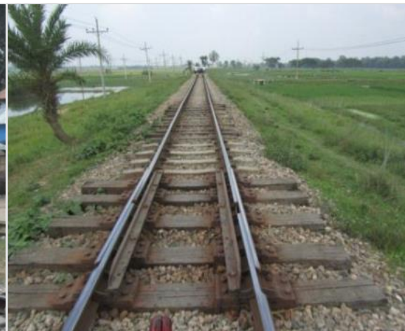
Photo 8: Switch Expansion Joint, Akhaura - Laksam Section
