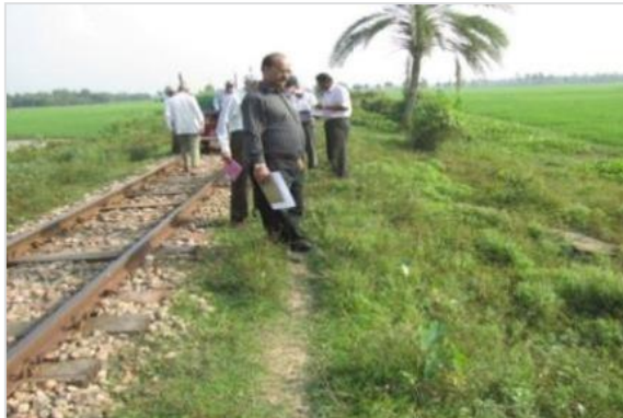
Photo 3: Soft soil, Akhaura-Laksam Track under Speed Restriction
