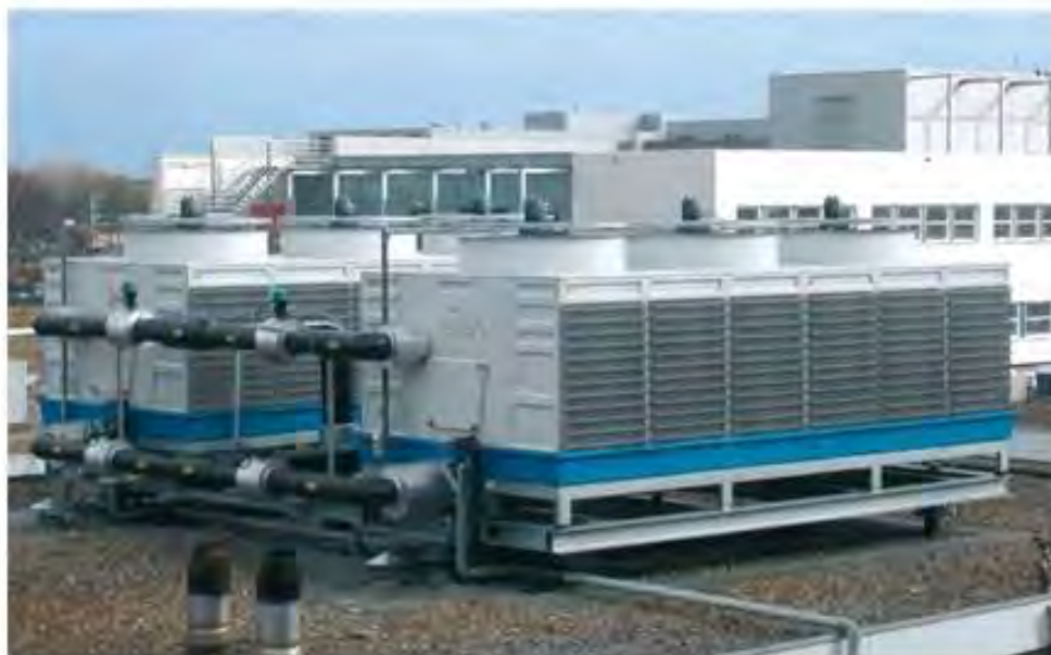
Figure 1.3.5.-4. The counter-flow cooling tower - "Low noise" performance achieved by fitting a large axial fan with speed control
