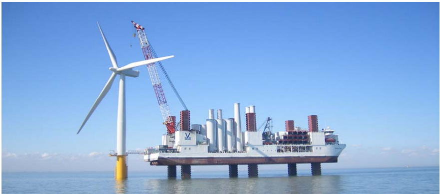
Turbine construction using jack-up barge (MPIO Resolution)
