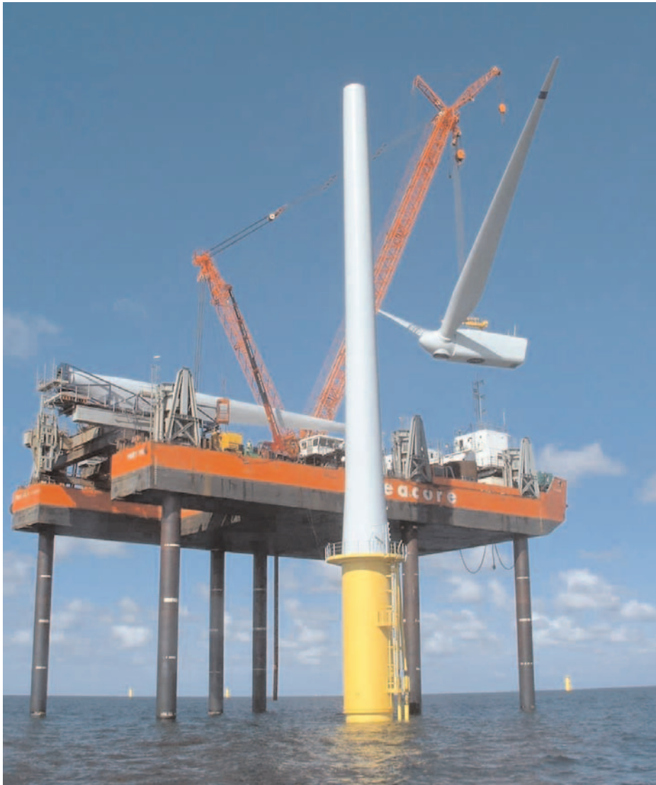
Figure 6 Installation of turbine nacelle using a jack-up barge
