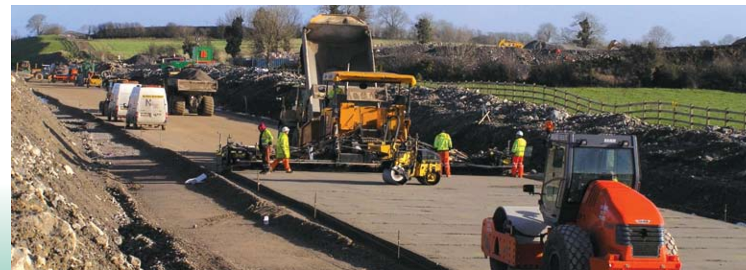
ROAD CONSTRUCTION WORKS
