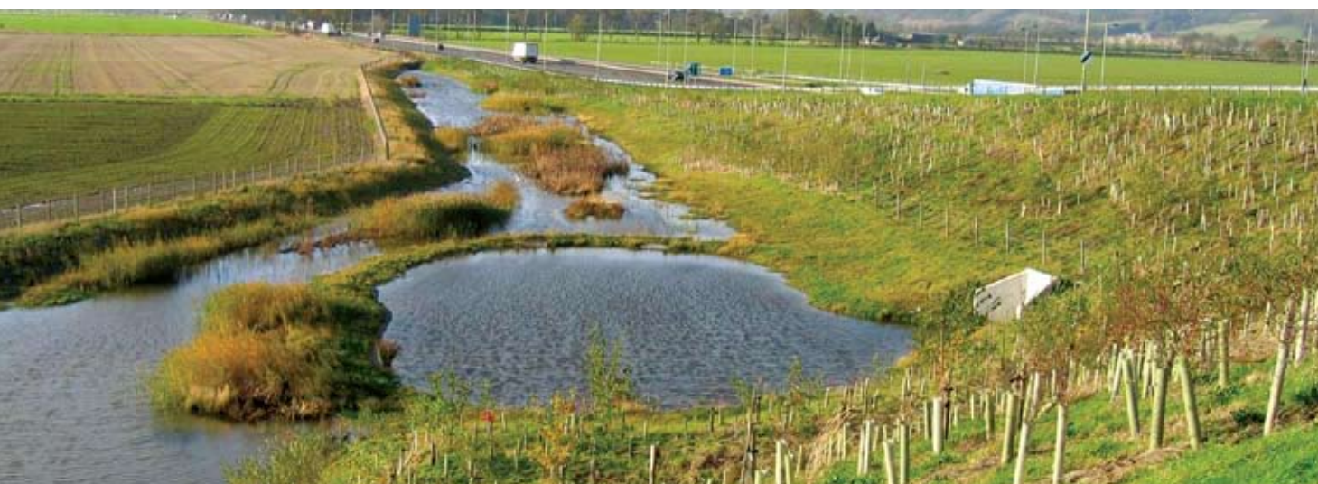
EXAMPLE OF DRAINAGE PONDS
