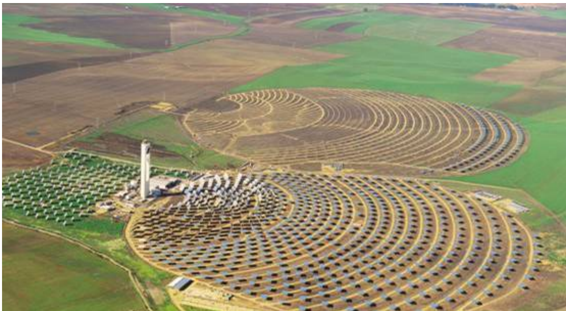
Figure 2: Power tower and heliostat field which is part of Abengoa Solar's Solúcar Platform in Sanlúcar la Mayor, Seville (Spain) 2 .
