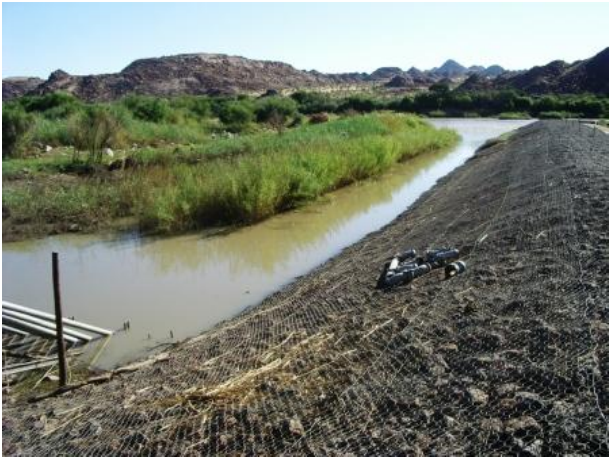
Figure 5.10: Man-made channel and upstream berm at the existing site of abstraction at Raap en Skraap.
