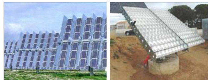
Figure 1.3: Low (left) and high (right) concentration PV plant trackers (source: !KaXu CSP Solar S.A., 2008)
