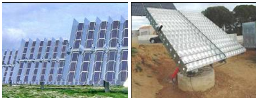
Figure 1.5: Concentrating and tracking PV (source: !KaXu CSP Solar S.A., 2008)
