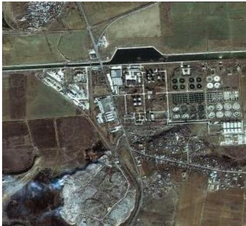
Fig. 4.8 WWTP position in connection with the Glina village and Ochiul Boului landfill
