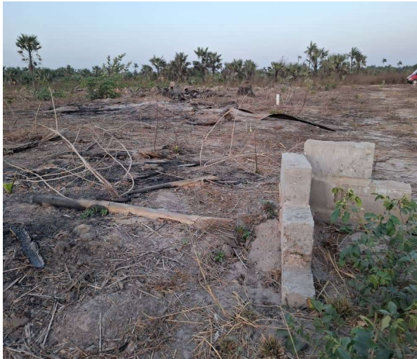
Figure 30 : Start of construction on borehole BHF9 site
