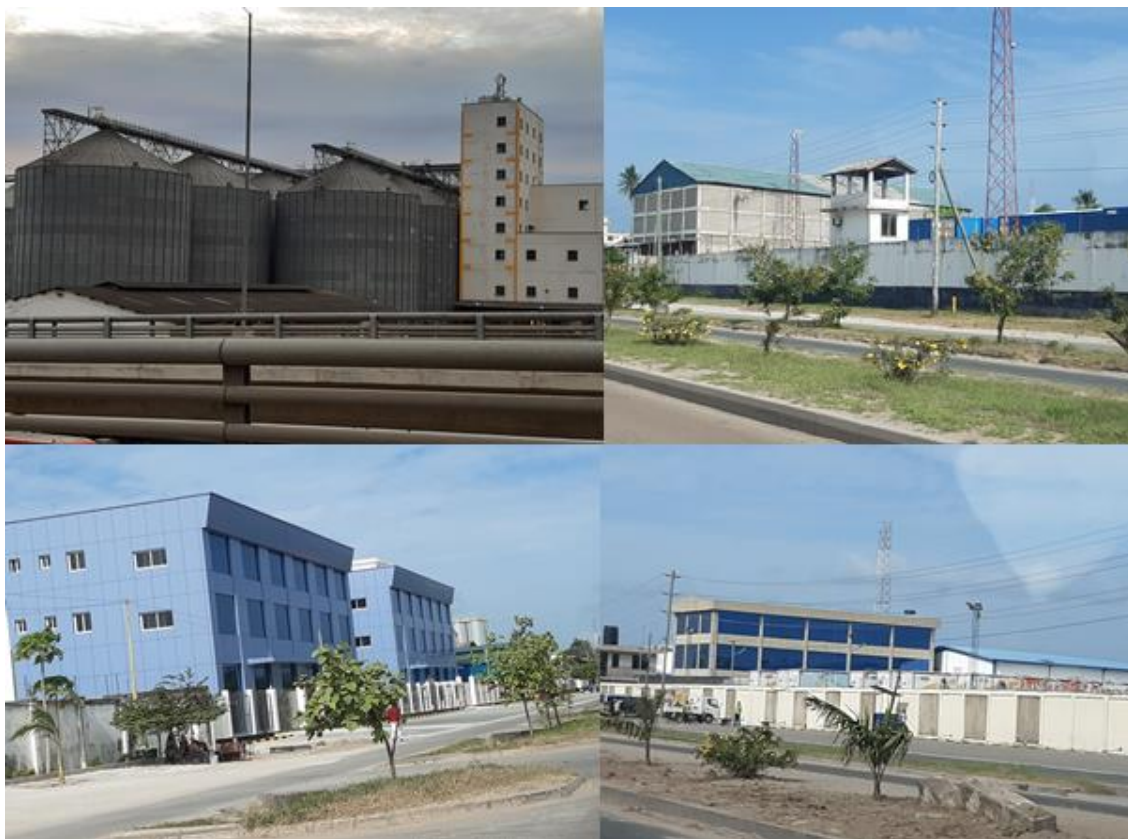
Figure 4-25: Industrial establishments along the BRT Phase 5 RoW Source: Consultant, July 2020
