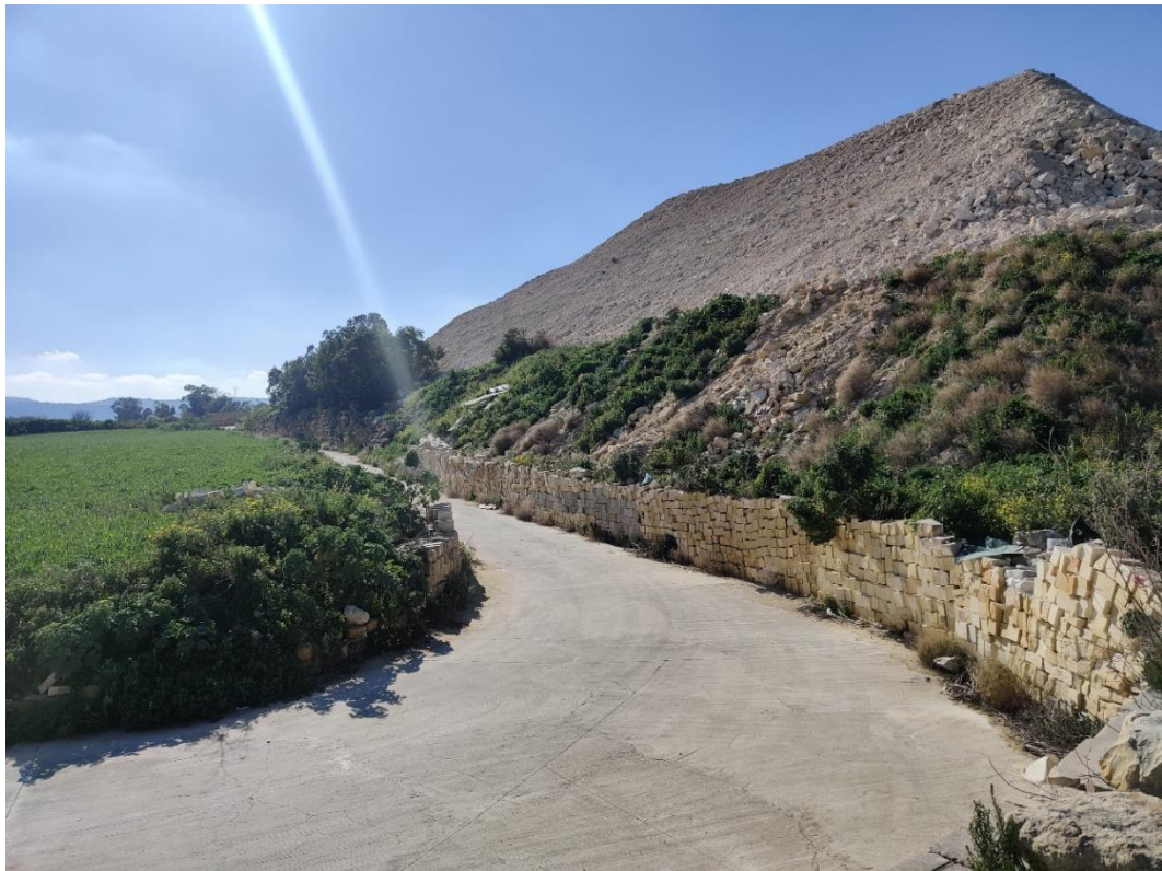
FIGURE 6: CONCRETE ROAD PROVIDING PUBLIC ACCESS TO THE NEARBY BOATYARD AND FIELDS (21 ST FEBRUARY 2023)
